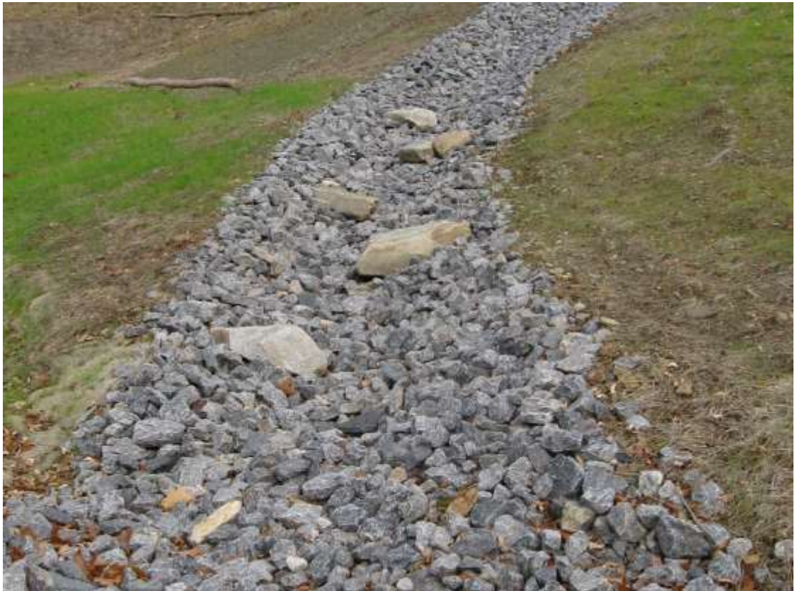
Fig.5. riprap erosion control
