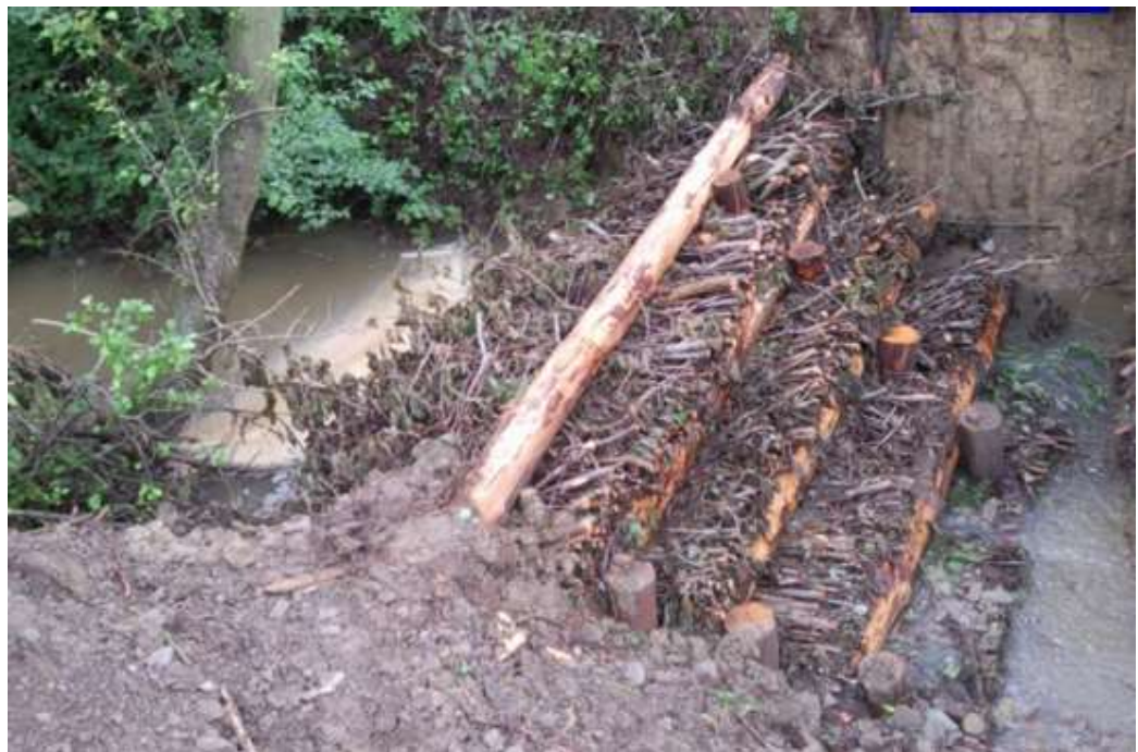
Fig. 9.sediment capture ponds
