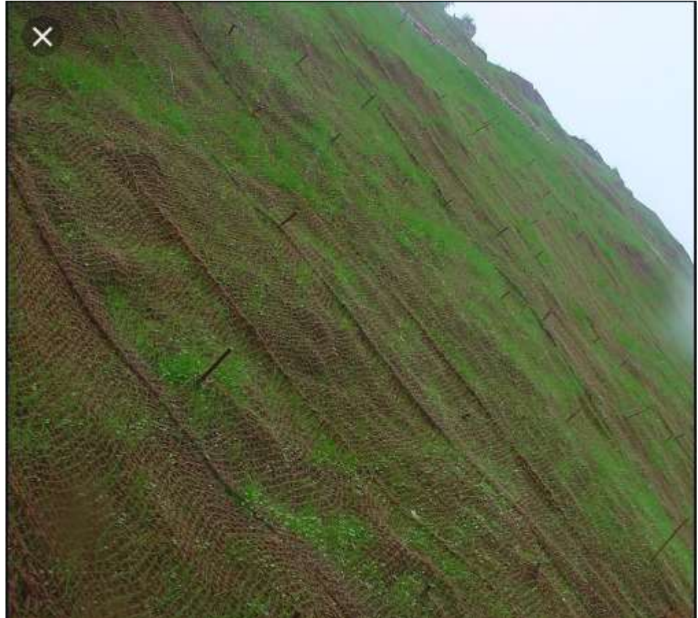
Fig.3. matting erosion control
