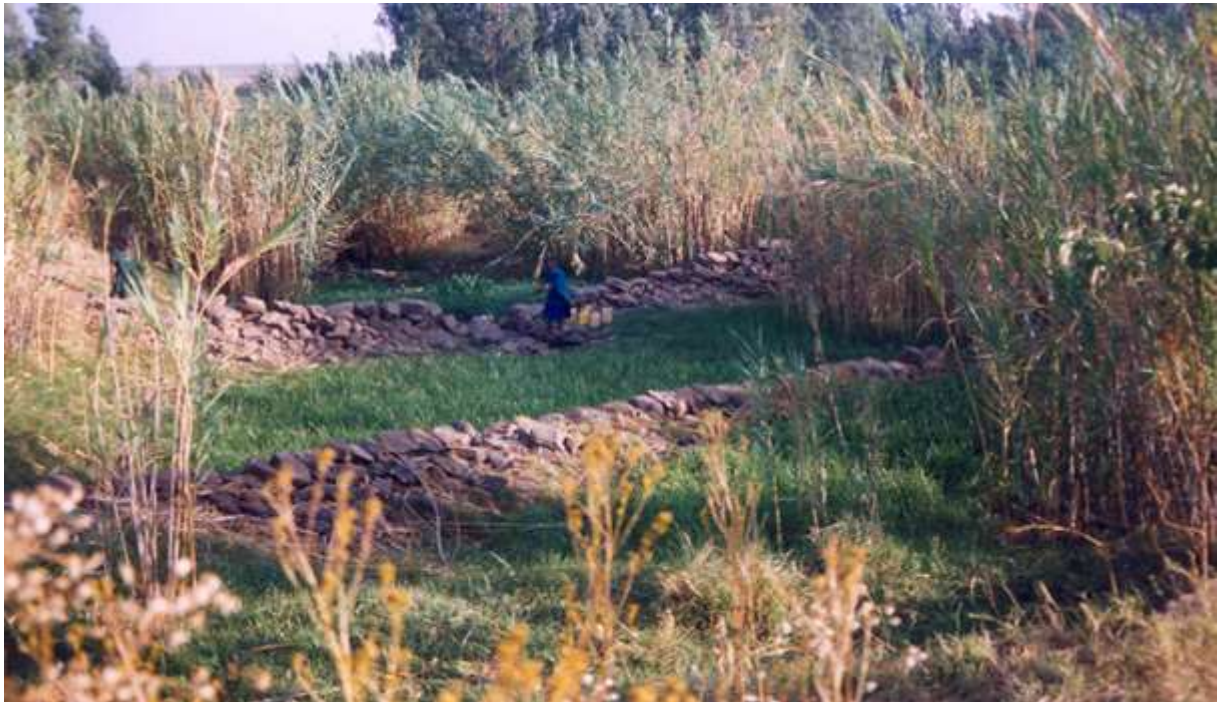
Fig.8. stone check dams
