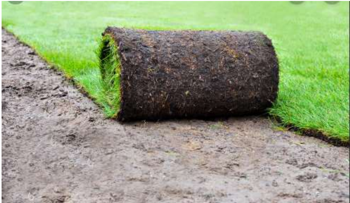
Fig.2. sodding erosion control
